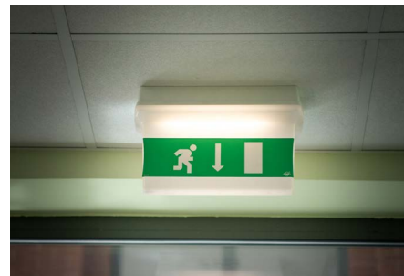
Measurement of emergency and evacuation lighting
